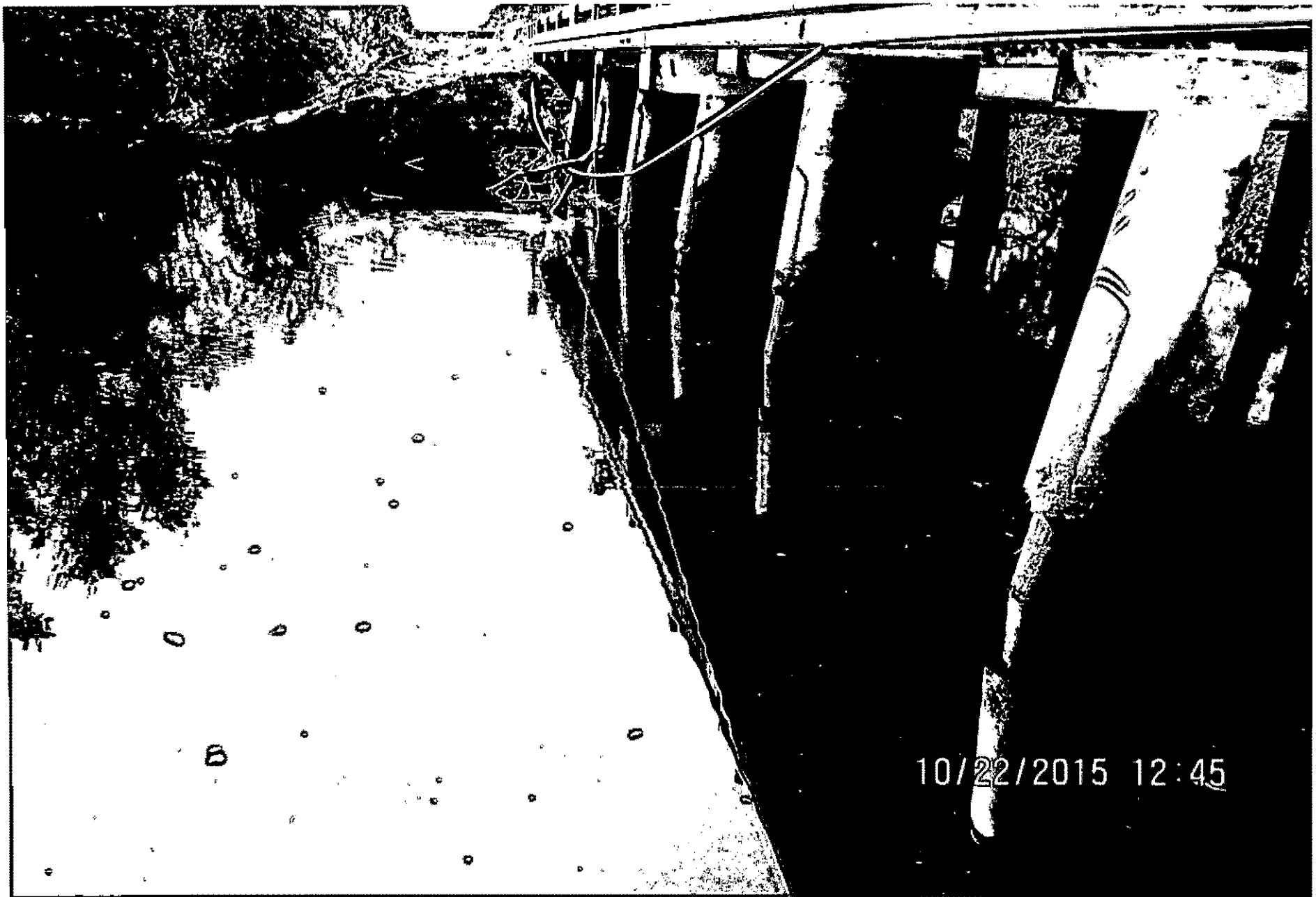
14-2-00301-0-13-00 Scour of Streambed & Washing of Slope Protection under Beginning of Bridge
